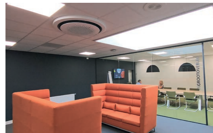
Office Building Edam, The Netherlands
